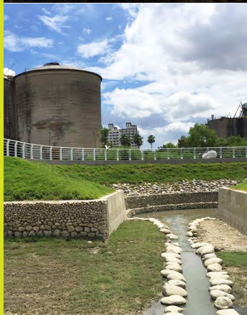
Shoushan Detention Basin Bypass Channel
