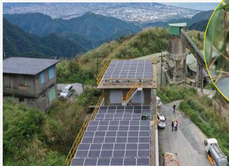
The Photovoltaic Energy Storage System at the Suao Taibaishan Mine
